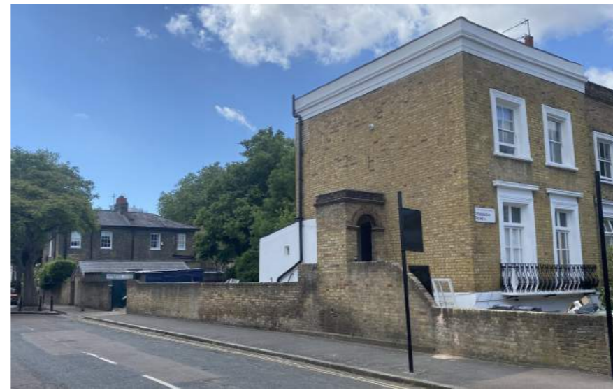
D) View of site and No.64 from Middleton Road
