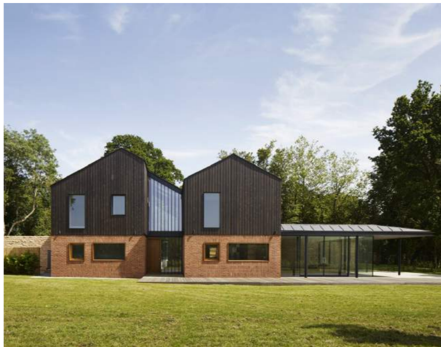
Split House, Windsor, Berkshire
